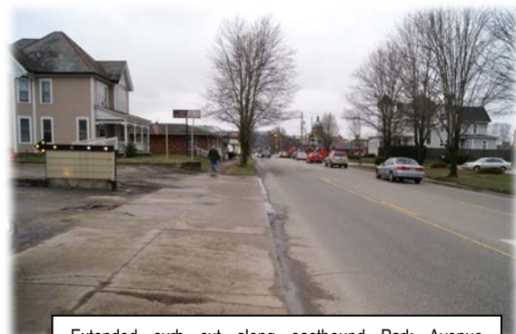
Extended curb cut along eastbound Park Avenue approaching 8 th Street (Century 21)
