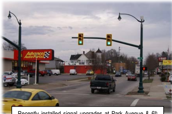
Recently installed signal upgrades at Park Avenue & 6 th Street
