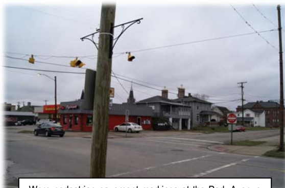
Worn pedestrian pavement markings at the Park Avenue & 7 th Street intersection
