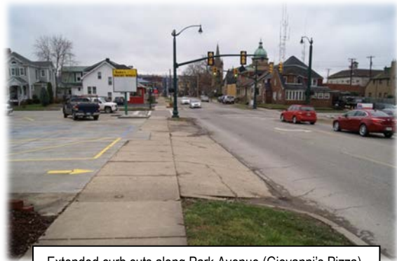
Extended curb cuts along Park Avenue (Giovanni's Pizza)
