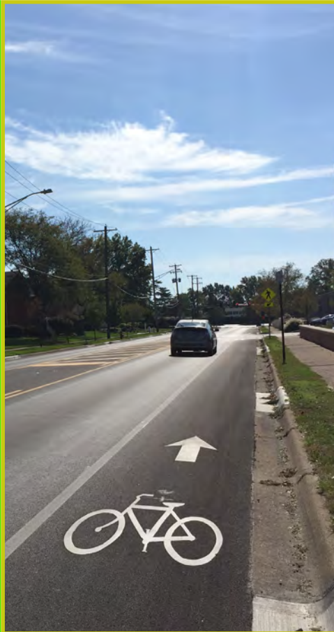
Figure 4.2: Visually Separated Facility
