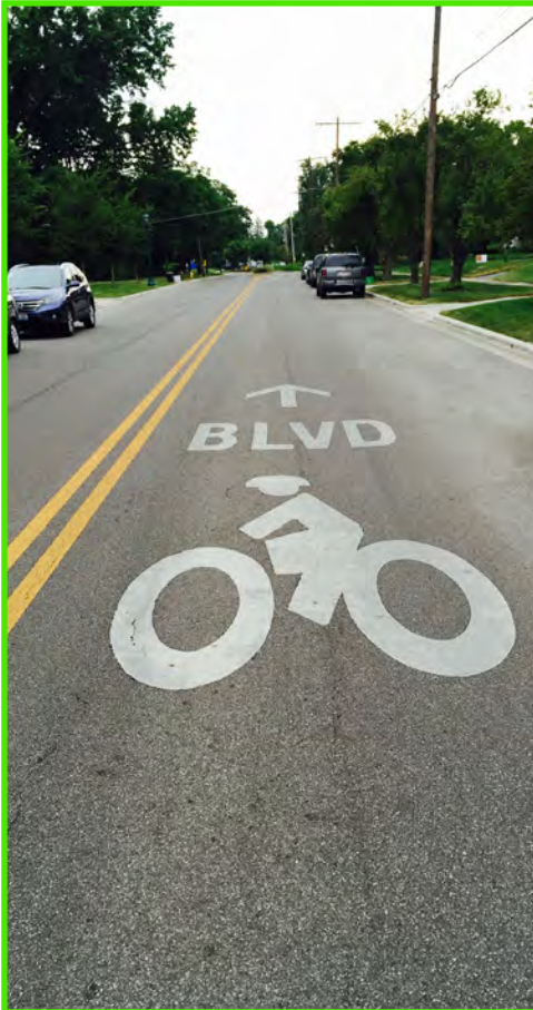
Figure 4.1: Mixed Traffic Facility
